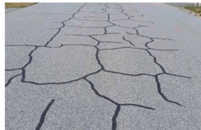
An interim crack sealing, - preventative maintenance, to extend the life of the asset (Fleet St - Access Road)
