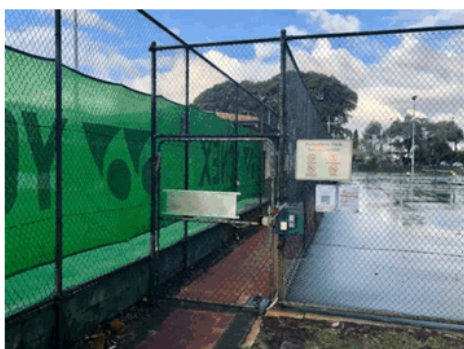
The existing entrance to the sports centre.
