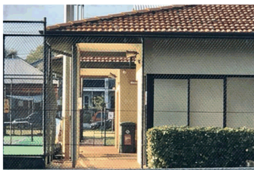
The arcade in front of the former sports shop which would become the new entrance to the sports centre (but without the link-mesh fence in front).
