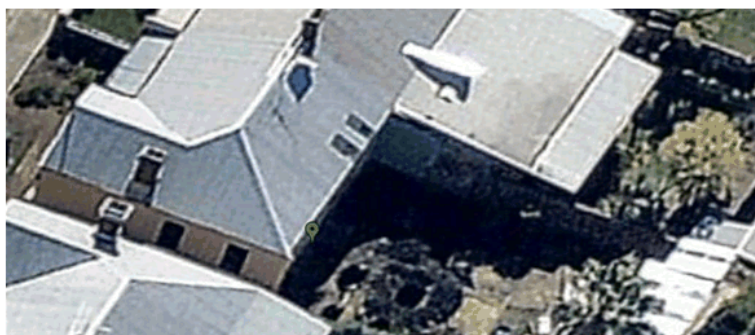
No.18 Moir Street After Demolition of Rear Skillion (August 2017)
