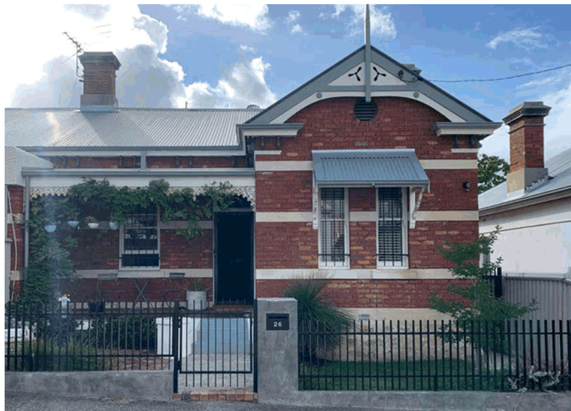
26 Moir Street Conservation Works (completion)
