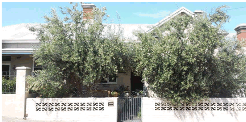
26 Moir Street Conservation Works (before)
