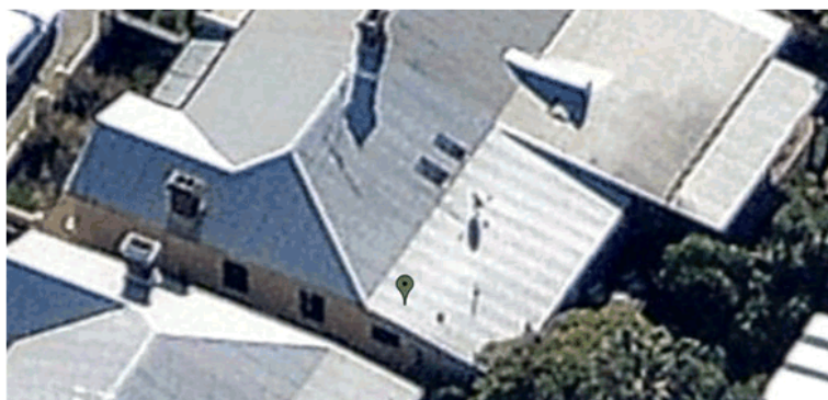
No.18 Moir Street Prior to Demolition of Rear Skillion (June 2017)
