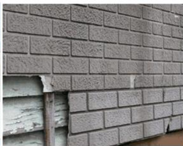
False brick cladding
