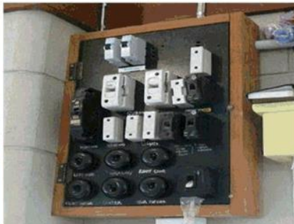
Electrical Switchboard and ceramic fuses
