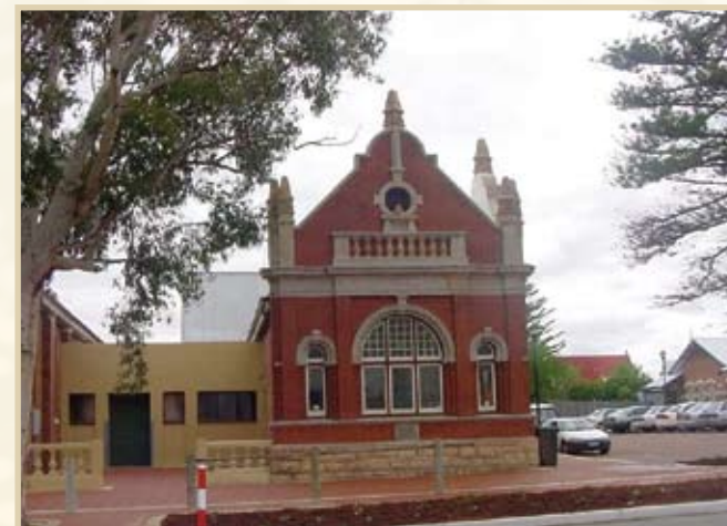
North Perth Town Hall Lesser Hall, built 1902 (2000)
