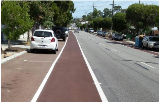
Figure 1. Sample view of existing Bulwer Street unprotected bike lane
