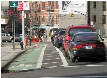
Figure 4. Example of bike lane protected by parked cars (painted in this case)
