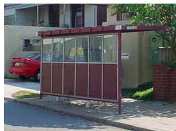
Cantilever style shelter
