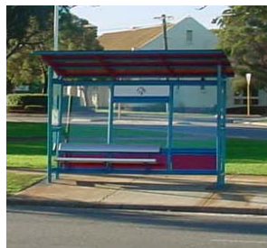
JSc style shelter
