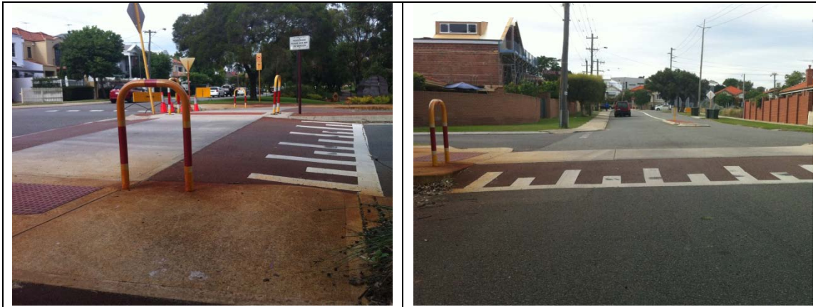
Existing raised plateau on Bourke Street, North Perth at Smiths Lake/Charles Veryard Reserve
