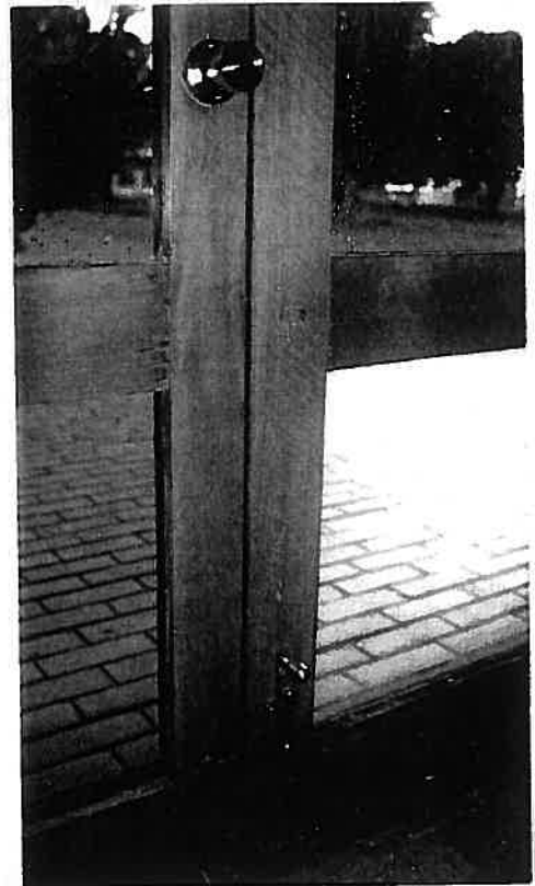
Photograph 55 Halvorsen Hall North east court doors. Interior view.
