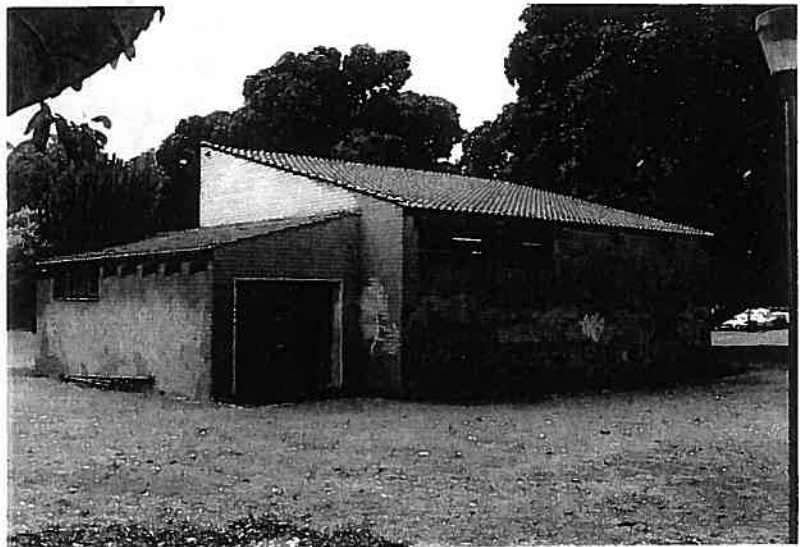
Photograph 44 Halvorsen Hall North west walls.
