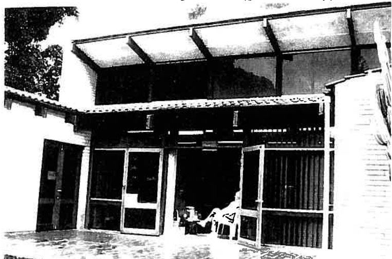
Photograph 41 Halvorsen Hall Clerestory windows on north east frontage.
