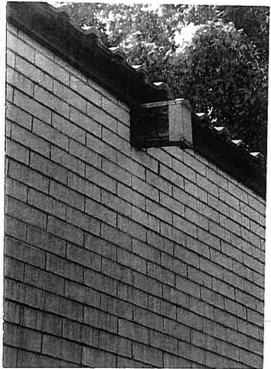
Photograph 43 Halvorsen Hall Rafter detail (south west wall)
