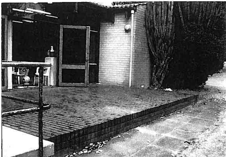
Photograph 48 Halvorsen Hall North east front -paved court.
