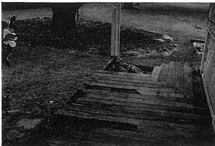
Photograph 24 Lee Hop's Cottage North east verandah.
