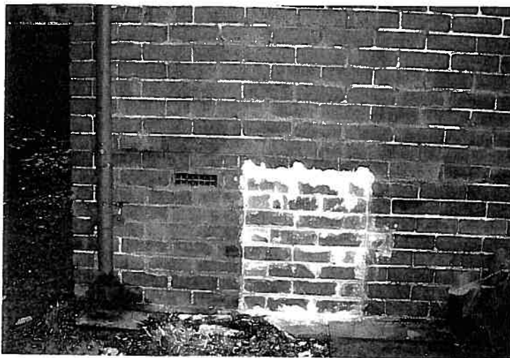
Photograph 22 Lee Hop's Cottage Rear repairs to 1975 brick wall.
