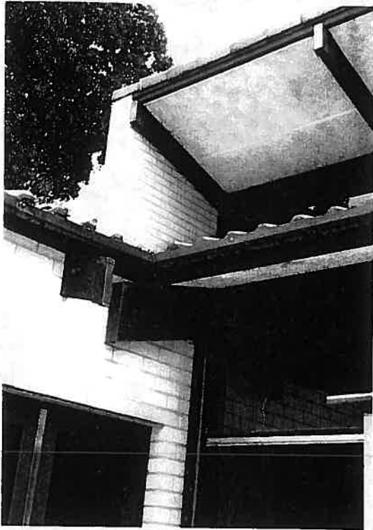
Photograph 42 Halvorsen Hall Roof and rafter detail (north east)
