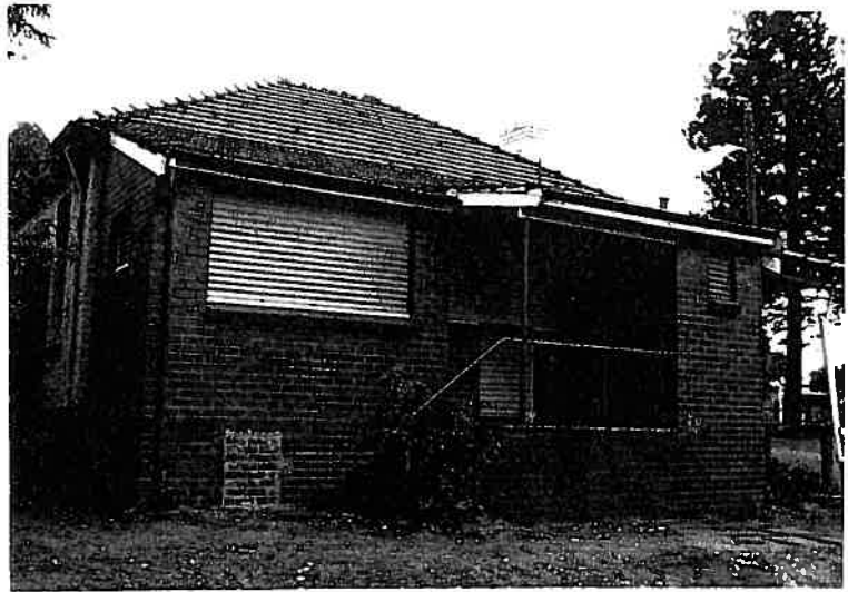
Photograph 33 Lee Hop's Cottage Rear verandah windows sheeted over.
