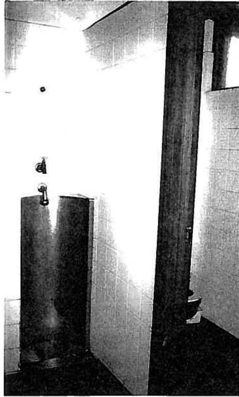
Photograph 52 Halvorsen Hall Mens Toilet.
