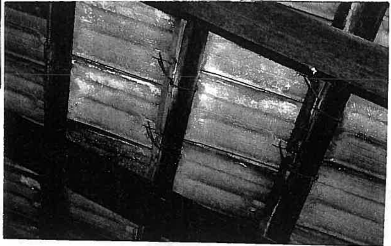
Photograph 13 Lee Hop's Cottage 1955 wired clay roof tiles.
