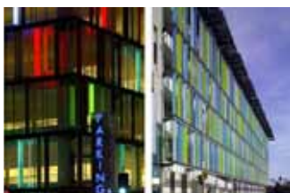
Screening devices, colour and lighting should be used to provide interest and break up the car parking building.
