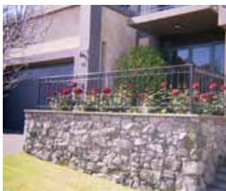
Open style fencing helps create a friendly neighbourhood and increases security through passive surveillance.
