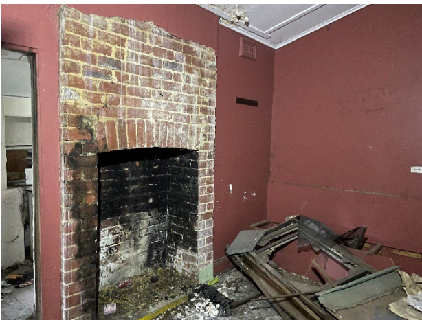
Figure 54: Dining Room (former kitchen)
