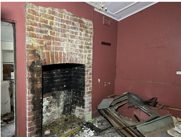
Figure 29: Dining Room (former kitchen)
