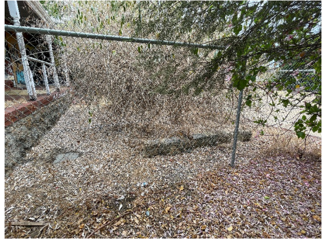
Figure 35: Fenced western side of the lot and some remnant hardscaping.
