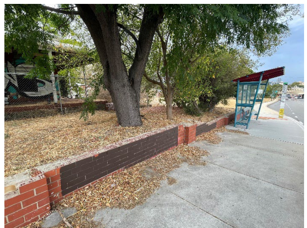
Figure 17: View showing relationship to Guildford Road.
