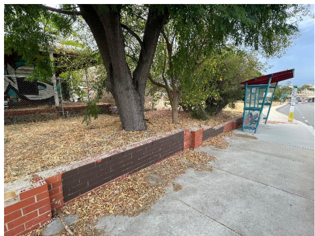
Figure 17: View showing relationship to Guildford Road.
