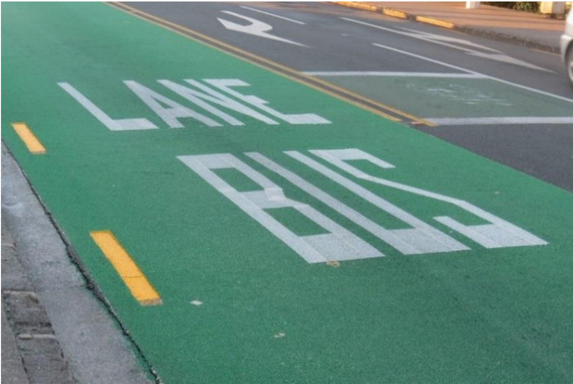
Figure 8.2: Example of the green coloured bus facilities used in New Zealand
