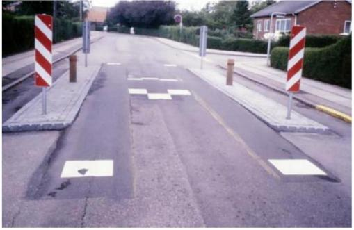
Combination road humps such as the example in Figure 8.3 have flatter ramps for buses straddling more severe plateau ramps for general traffic (Kjemtrup 1988). Note also provision for cyclists to bypass the narrowed section.
