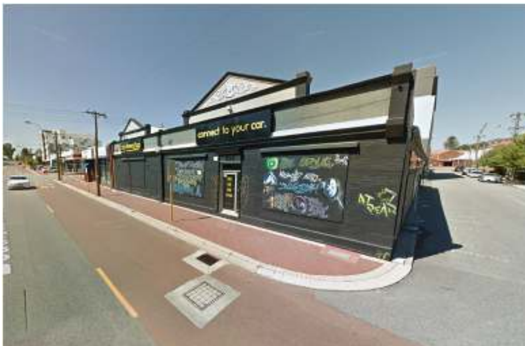
Figure 1 – Subject site during previous occupation in March 2017 with boarded windows (Source: Google Street View)
