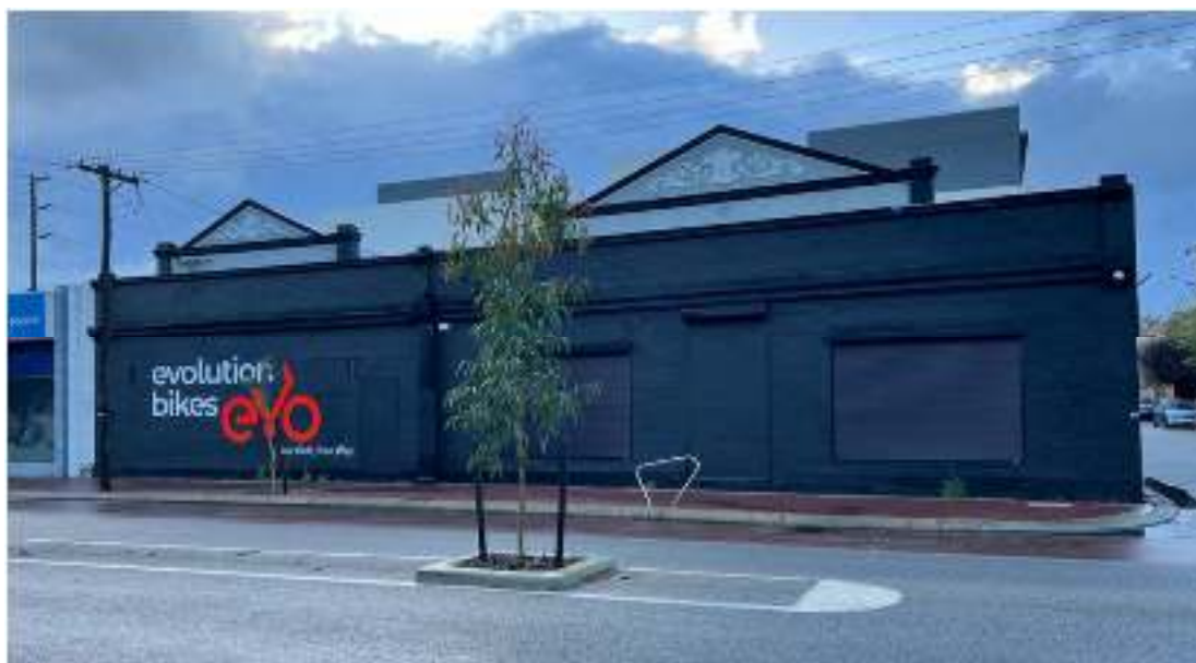
Figure 3 – Subject site with roller shutters closed.
