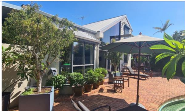
Rear two storey extension to eastern elevation
