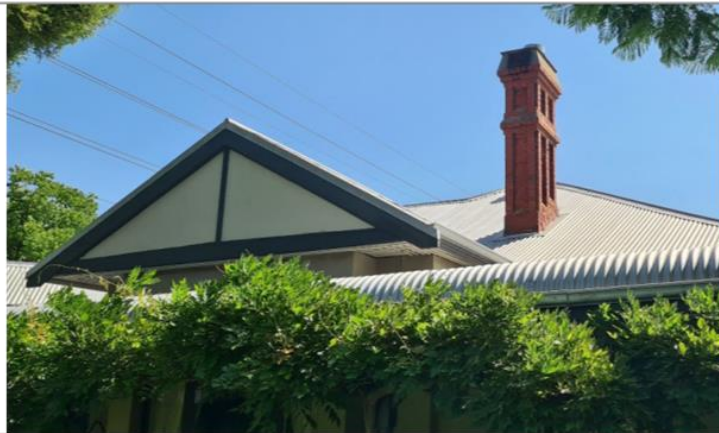
Gable and chimney to southern elevation
