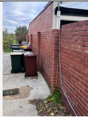
Photograph of wall prior to demolition 19 August 2022.
