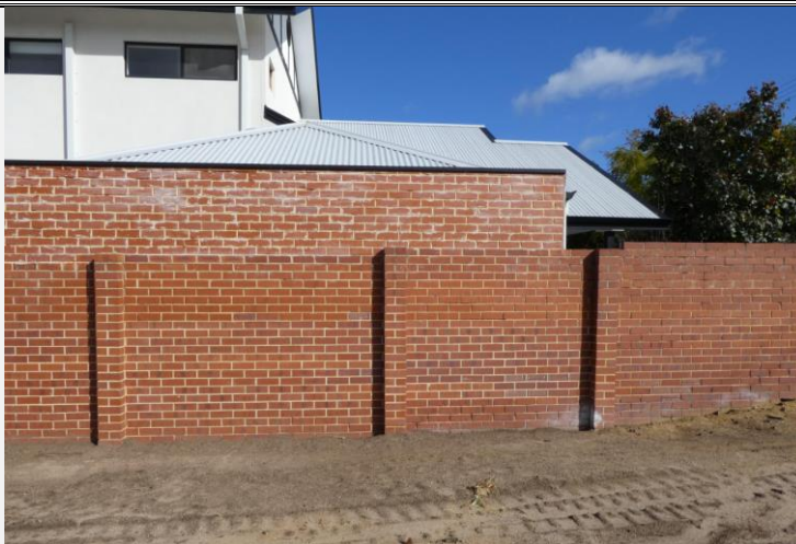
Photograph of wall after site works. 16 August 2023
