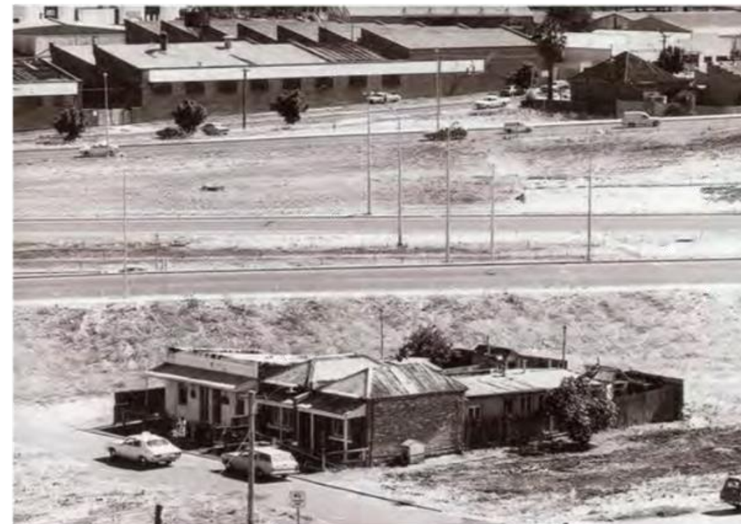
The construction of the Mitchell Fwy in the early 1970s saw the demolition of residences in Simpson Street, two of which still remain today. Credit: Andrew Kailis
