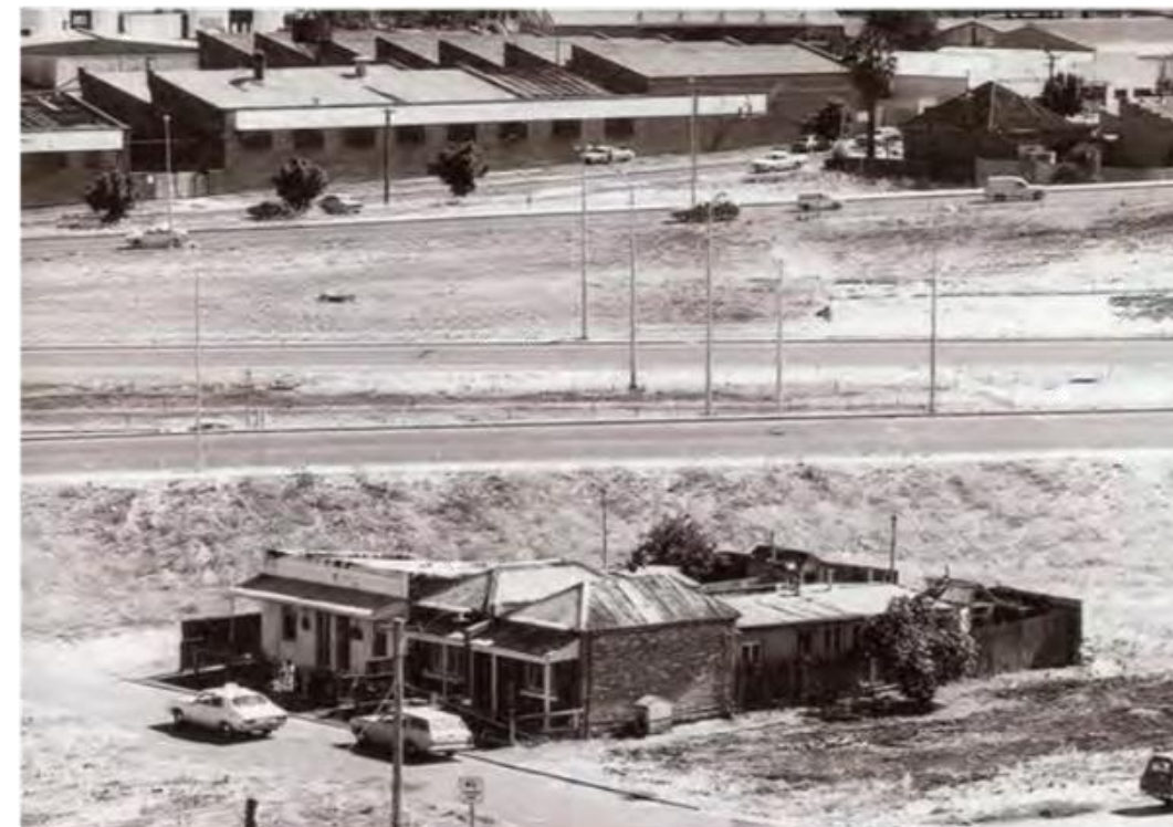
The construction of the Mitchell Fwy in the early 1970s saw the demolition of residences in Simpson Street, two of which still remain today. Credit: Andrew Kailis
