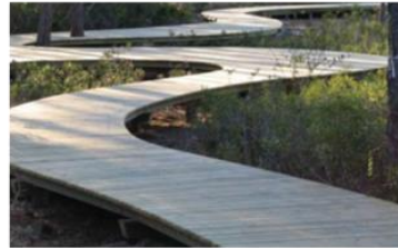
Figure 54. Example of raised timber boardwalk.
