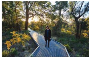
Figure 55. Raised perforated steel boardwalk.
