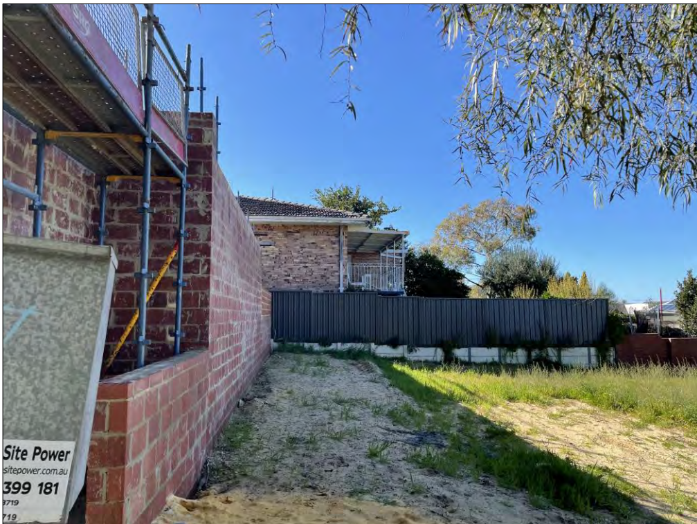
Image 2: An eastward view of the boundary wall and existing parapet wall between 31 Gill and 80 Auckland Street, in addition to the upper floor of 29 Gill Street.
