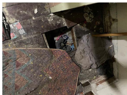
Figure 47: Detail of floorboards.
