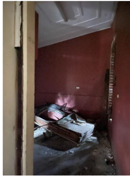
Figure 61: Sleepout looking through to Dining Room.
