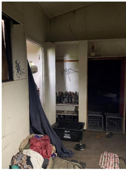
Figure 60: Sleepout looking through to Dining Room.
