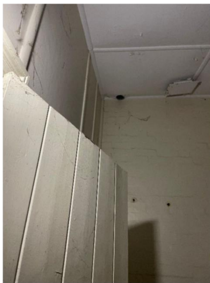
Figure 62: Bathroom door and ceiling.
