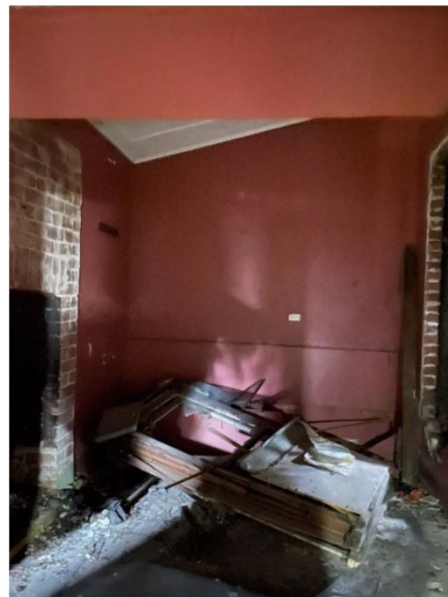
Figure 55: Dining Room (former kitchen)
