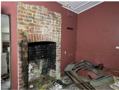
Figure 54: Dining Room (former kitchen)
