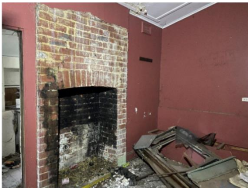
Figure 29: Dining Room (former kitchen)
