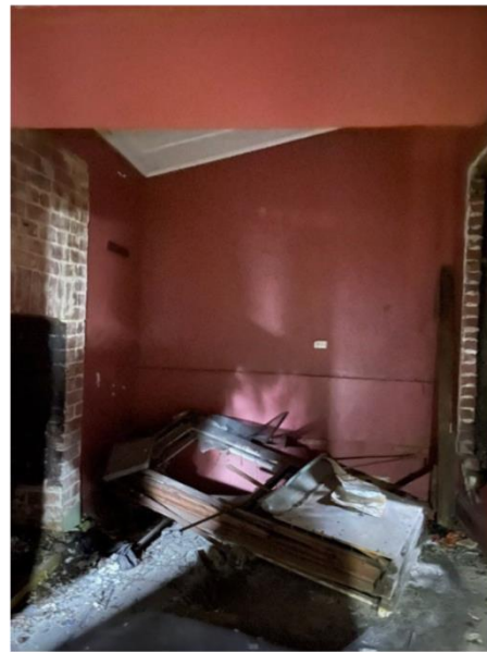
Figure 30: Dining Room (former kitchen)
