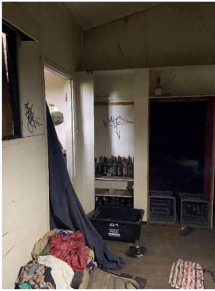
Figure 60: Sleepout looking through to Dining Room.
