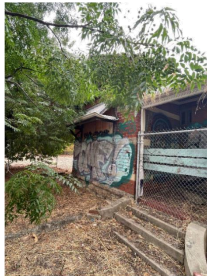
Figure 25: Front Elevation showing original steps.
