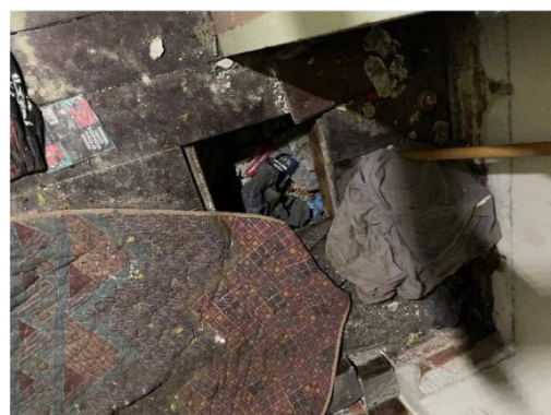
Figure 47: Detail of floorboards.
