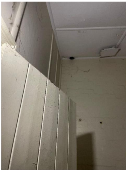
Figure 62: Bathroom door and ceiling.
