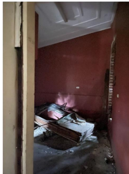
Figure 61: Sleepout looking through to Dining Room.
