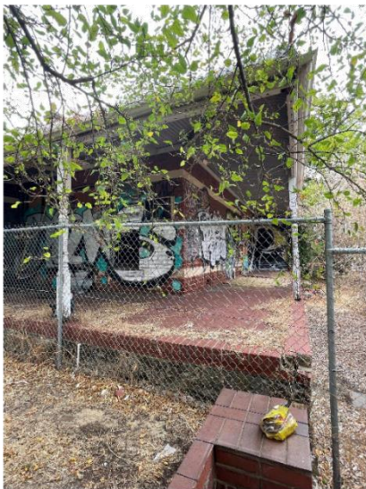
Figure 24: Front Elevation showing verandah.
