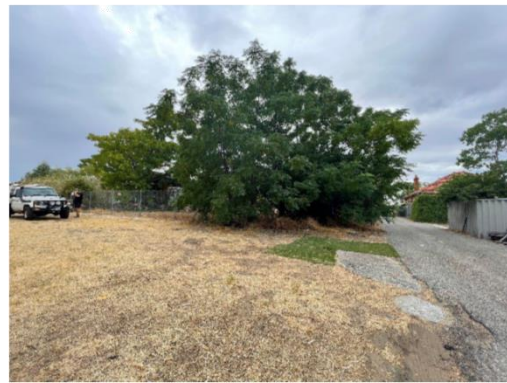
Figure 15: View from the lane to the western elevation.
