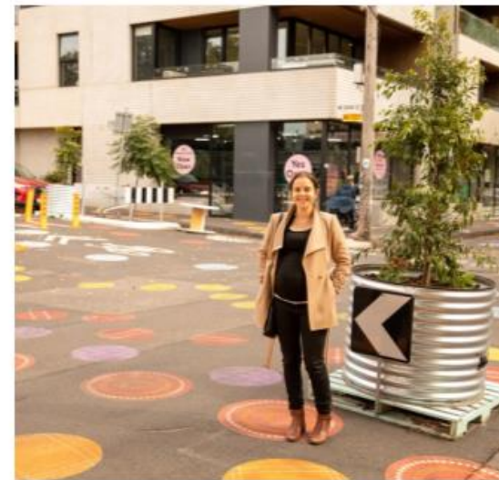
Painting road surface (water-based paint)
