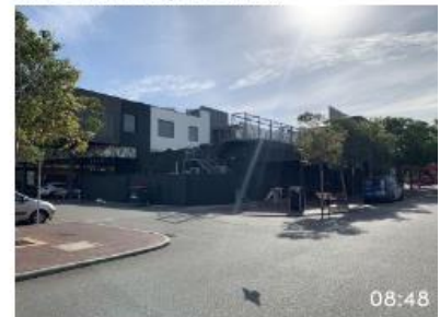
Back of The Elford bar facade
