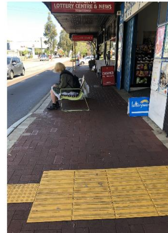
Bench at bus stop blocking access
