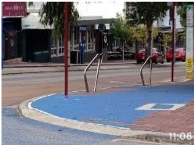
Bike rack very close to road on Beaufort Street.
