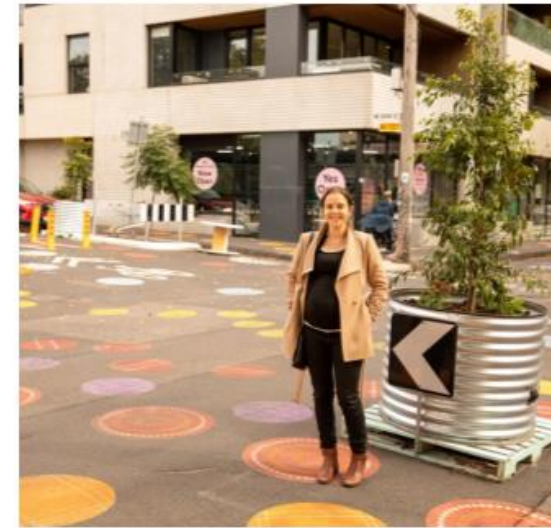
Painting road surface (water-based paint)
