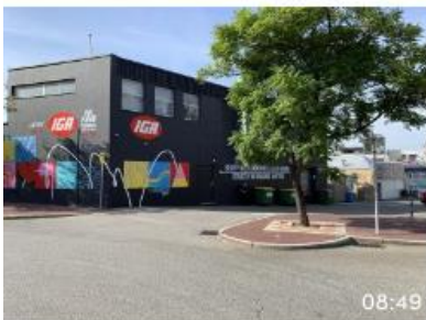
Back of IGA facade
