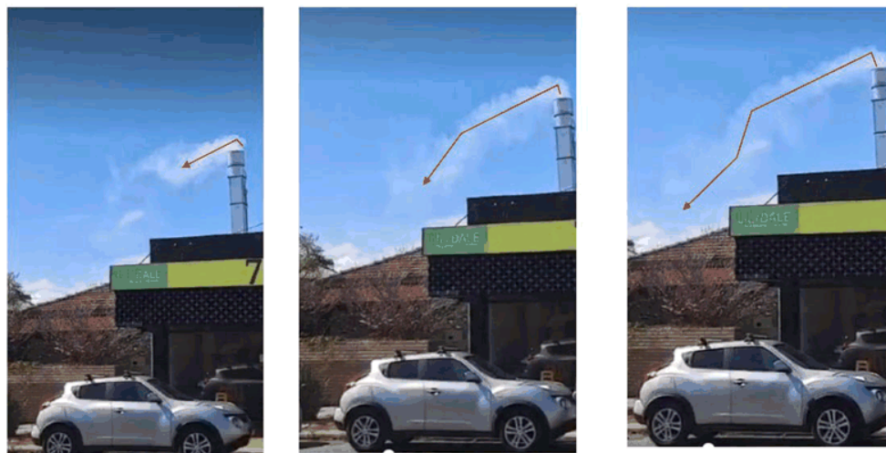
Figure 13: Sequence #1 – plume pushed down by downwash effect
