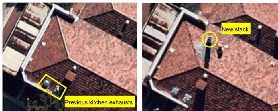
Figure 1: Former and new fume exhausts from the restaurant
