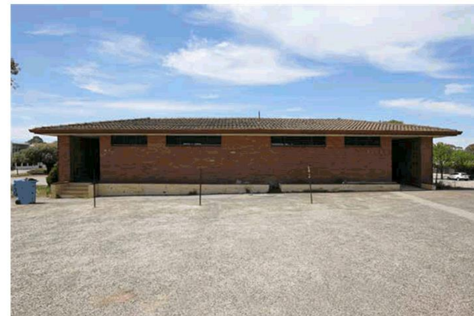
Existing toilet block
