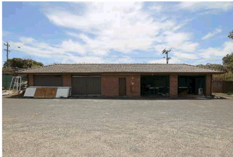
Existing Heritage Building
