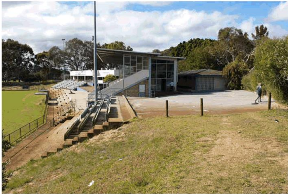
Existing Floreat Athena grand stand and toilet block - view from north
