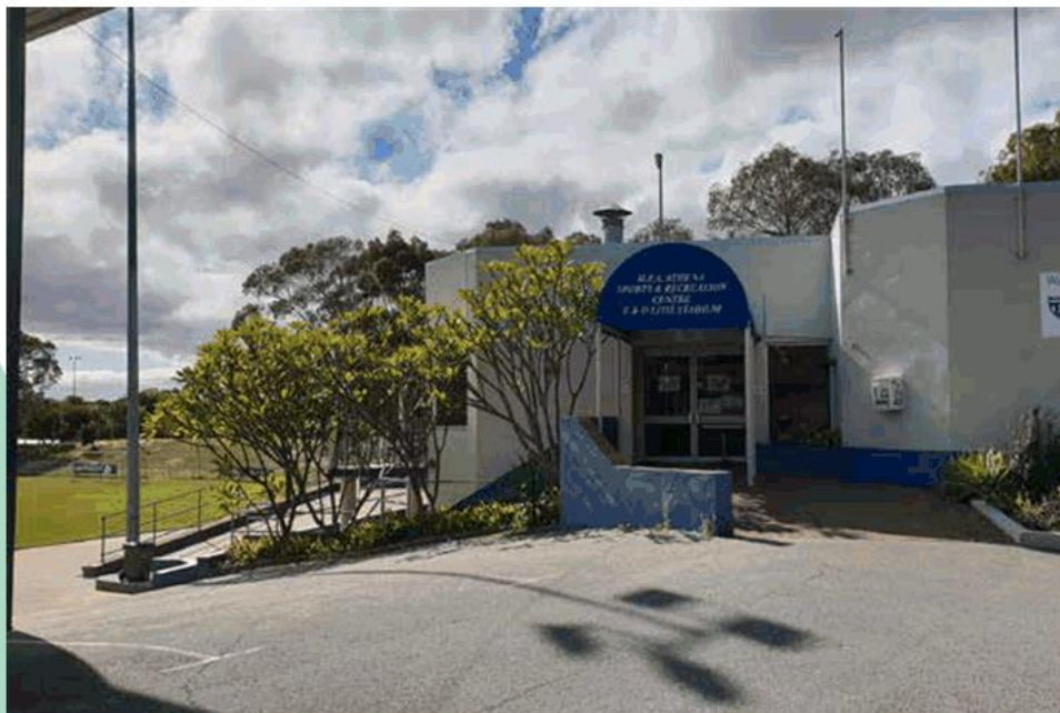
Existing entry to Floreat Athena Club
