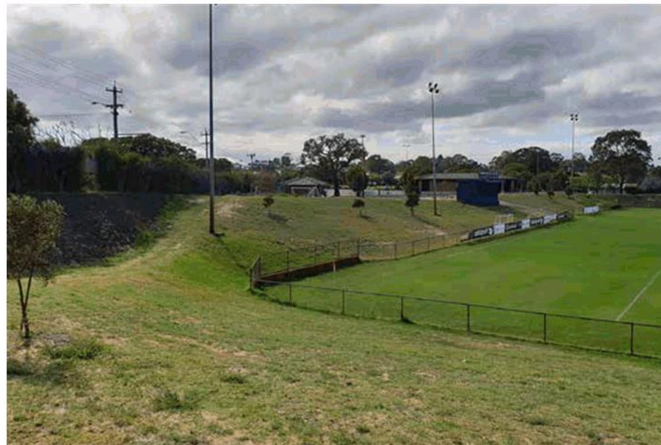
Northern edge condition of park looking east
