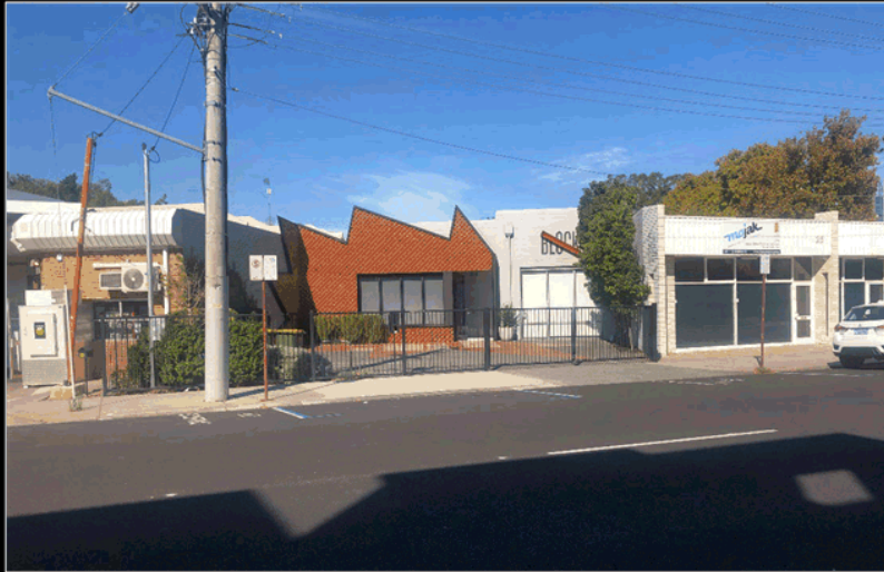
Existing conditions on south side of Brisbane Street, west of site
