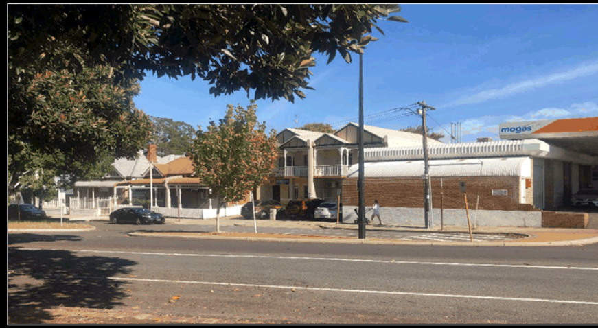
View of west side of Pier Street south of site
