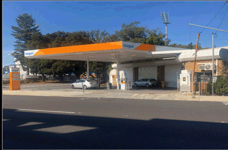
Existing site conditions – view from Brisbane Street south-eastwards across site
