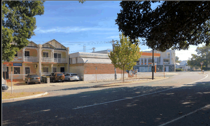
Existing conditions on Pier Street, south of site
